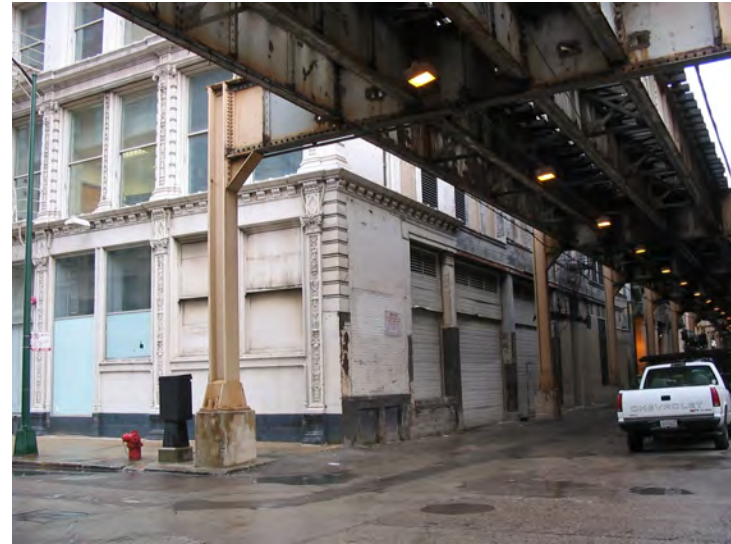
Alley (west) façade
