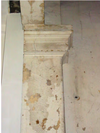
Detail of plaster wall and capital in the West Stairway
