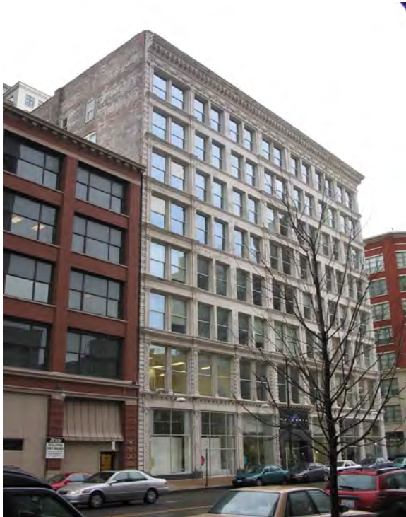
Portion of south façade (side wall) visible from street
