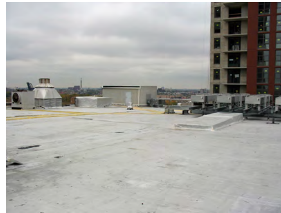
Roof view looking southwest
