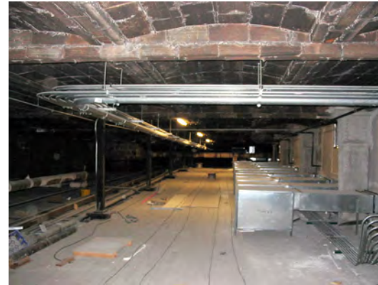
View of attic showing steel and clay-tile structure.
