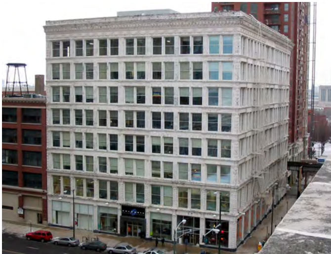
East and north facades
