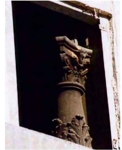
Remodeled Wabash Entrance (left) and inspection opening showing original terra cotta above entrance (right). Inspection opening (showing original terra cotta ornament behind granite) and photo by SAS Architects & Planners
