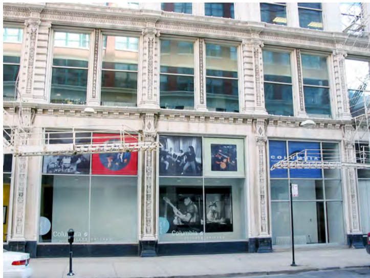
North façade, first and second floors
