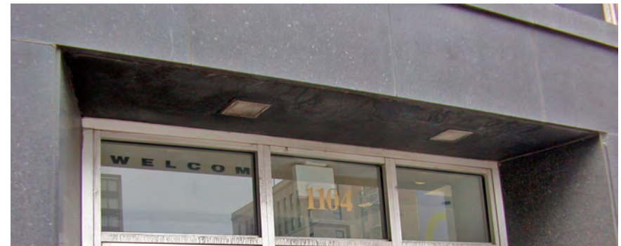
East elevation – incandescent downlights above east entry.
