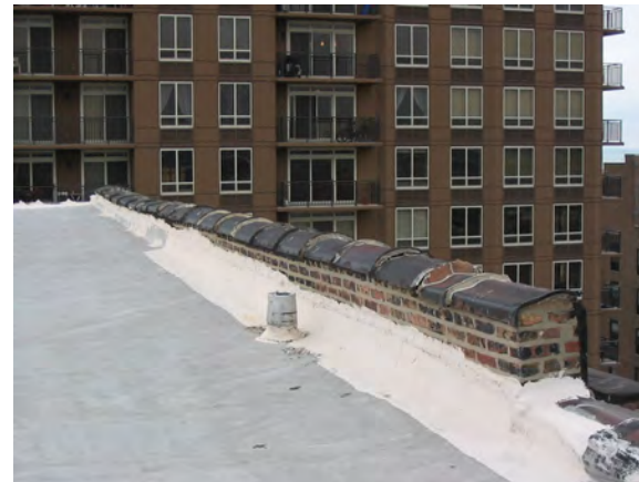
Portion of south parapet wall looking east
