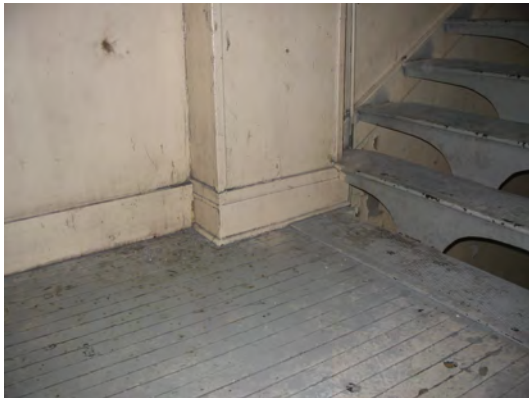
Detail of wood floor and wall trim at the West Stairway
