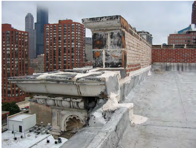
Edge of west parapet viewed from roof
