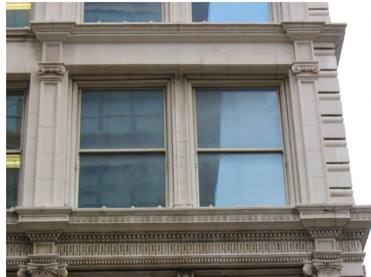
Upper floor façade detail
